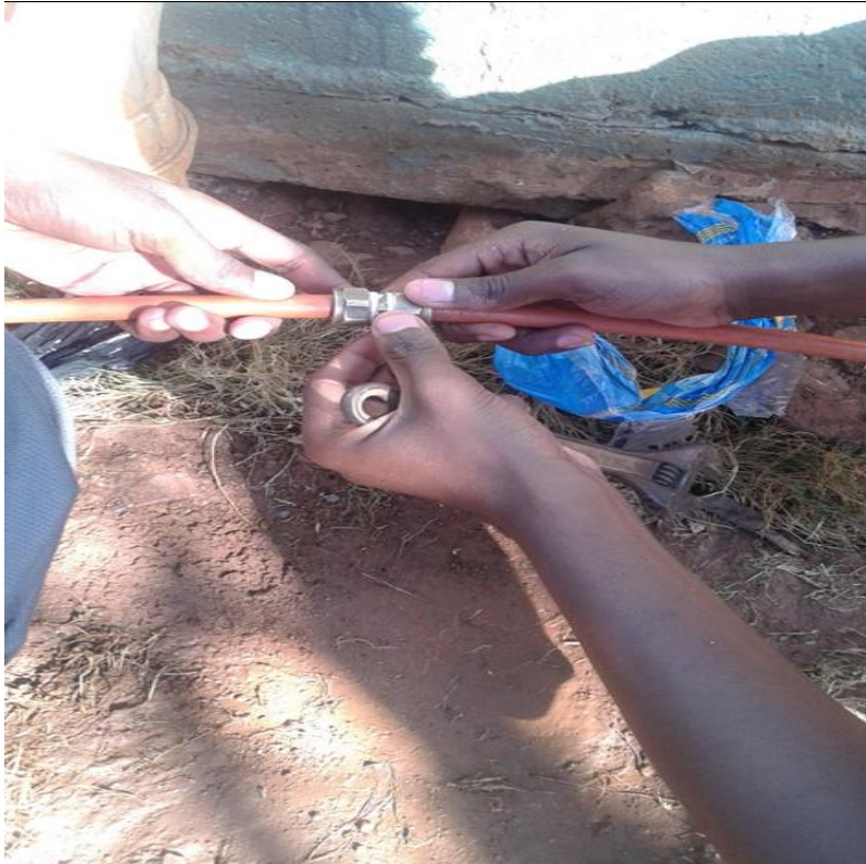
Figure 4.3b: The procedure of fixing a water leak ( source author )
