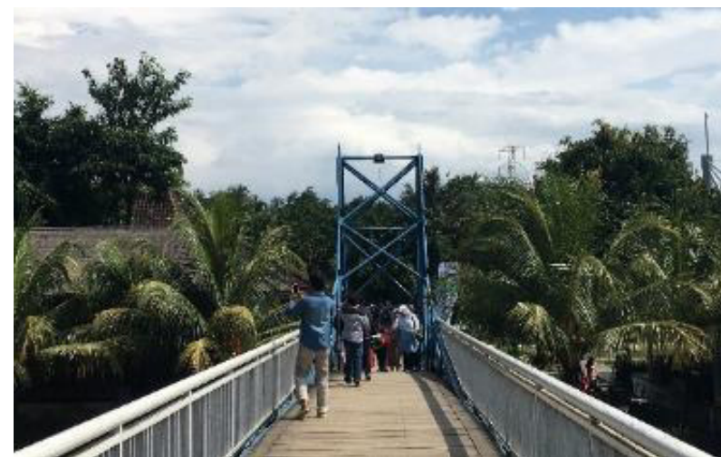
Gambar 37 / Figure 37: Kondisi dasar apung Ah Poong, Sentul Citu Condition in Ah Poong Floating Market, Sentul City
