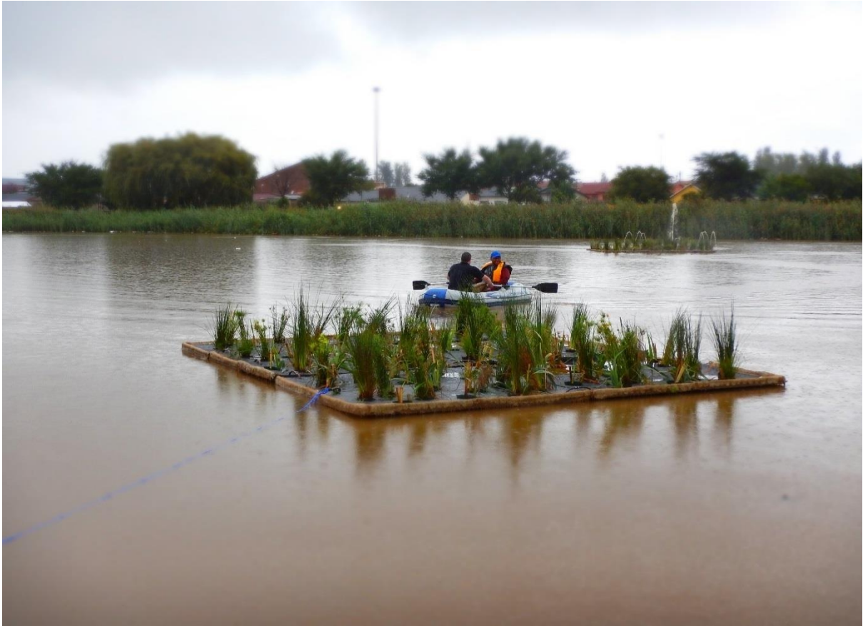
Figure 19: Installing two floating treatment wetlands on Moroka Dam, Rockville, Soweto (Photo: Yolandi Schoeman, Soweto, 17 March 2016)
