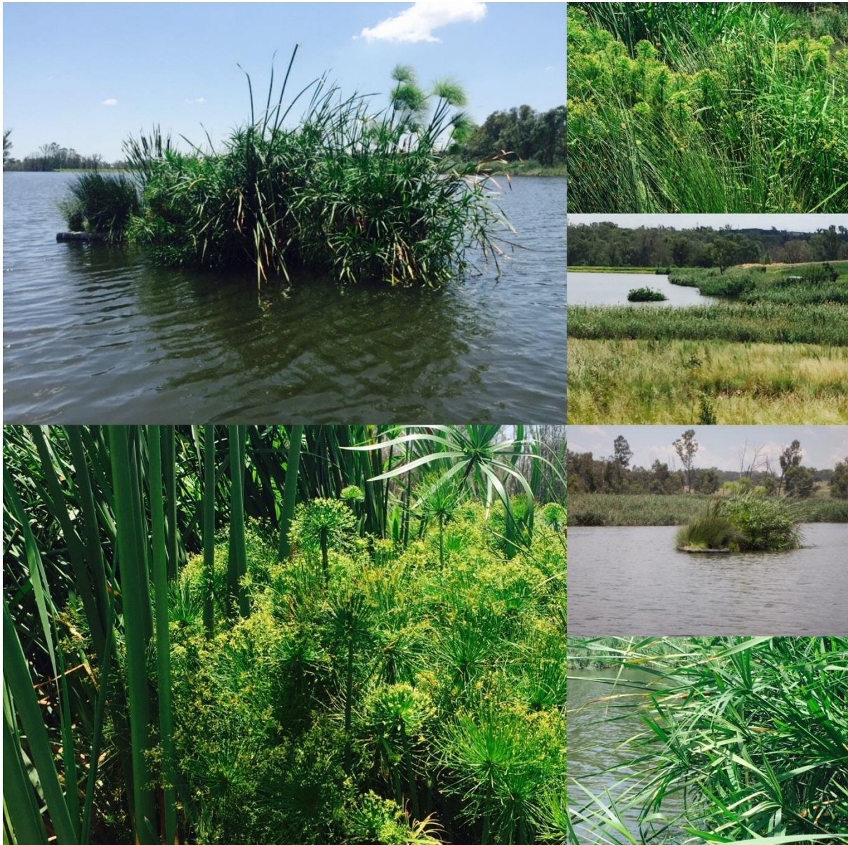
Figure 17: Floating treatment wetland islands installed at Modderfontein Nature Reserve, 2015 (Photo: Yolandi Schoeman, Modderfontein, 04 February 2016)
