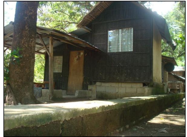
Figure 26. Elevated concrete path from the road to the house of a Papaya farmer
