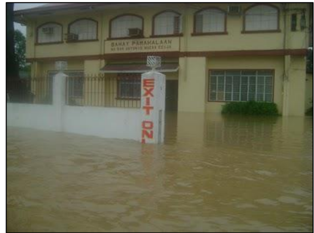
Figure 14. Flood in town proper of San Antonio, Nueva Ecija, Philippines, 2011
