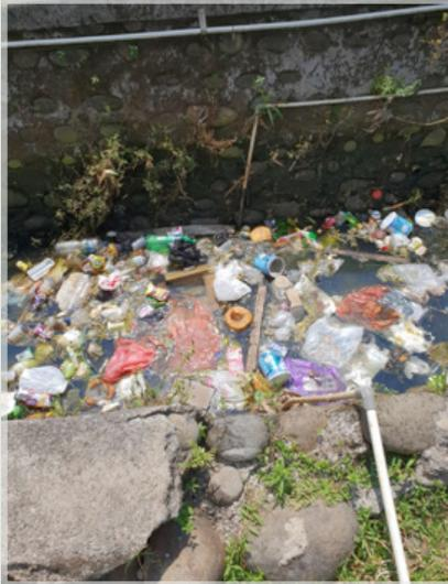
Fig. 3: Solid waste polluting and blocking waterways
