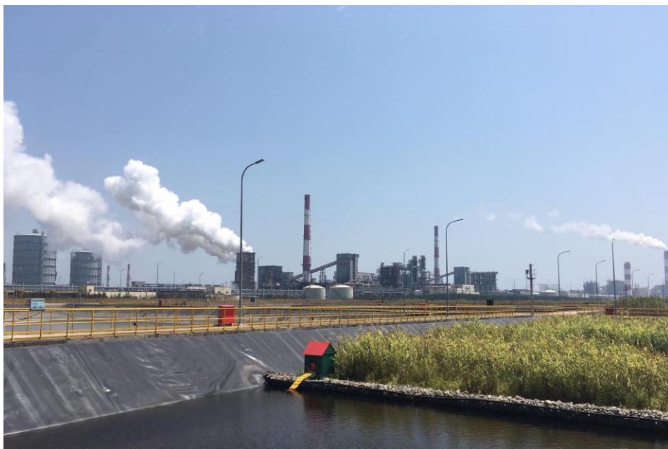
Photo 9.4: Formosa's Eco-park, with two furnaces of the thermal power plant (right) and the coking plant (central)
