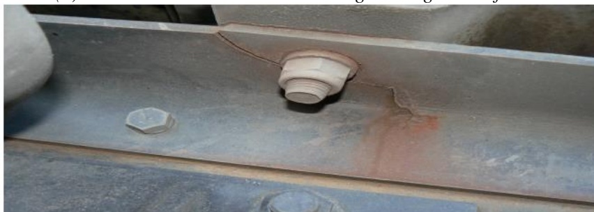
(b) A cracking at turntable ripple plate mount.
