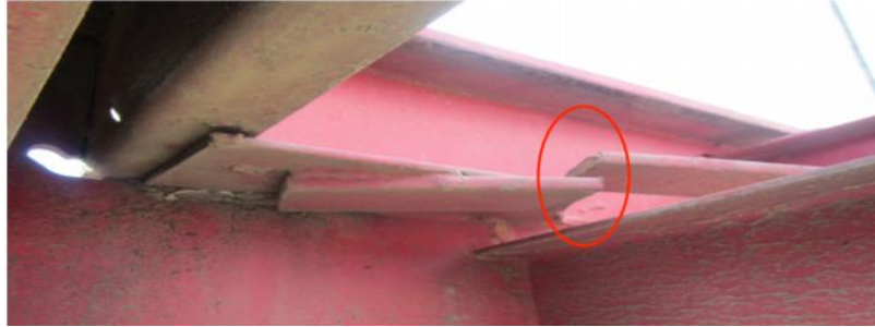
(c) Cracking at a log trailer cross support.
